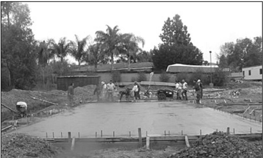
The concrete slab for the new building, just after being poured
