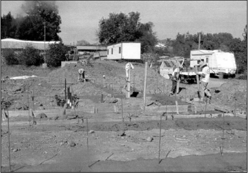
Preparation for the new foundation
