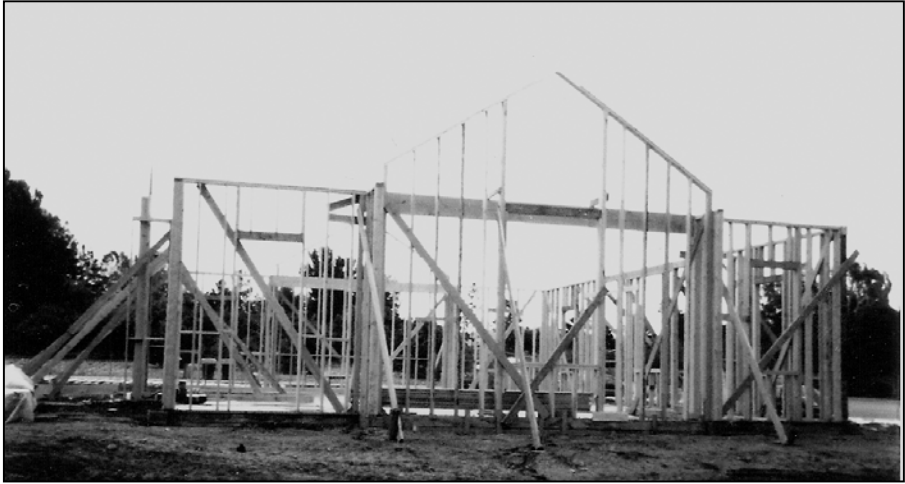
Framing begins on the new foundations
